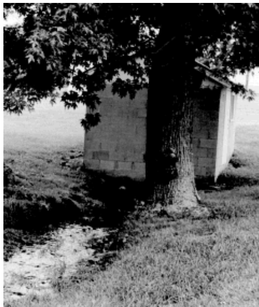
THE SPRING HOUSE AT DUG SPRINGS TODAY (For a view of an older version of the spring house, see Fern Angus's Down the Wire Road , page 21.
